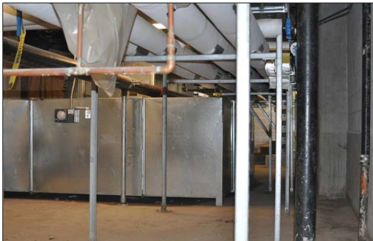
*Picture 5 - Basement area of the Center, taken February 23, 2011.
