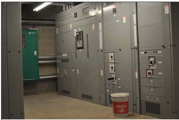
*Picture 3 - Basement area of the Center, taken February 23, 2011.
