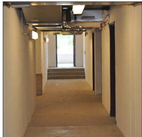
*Picture 6 - The Center basement exit door, taken June 1, 2011.
