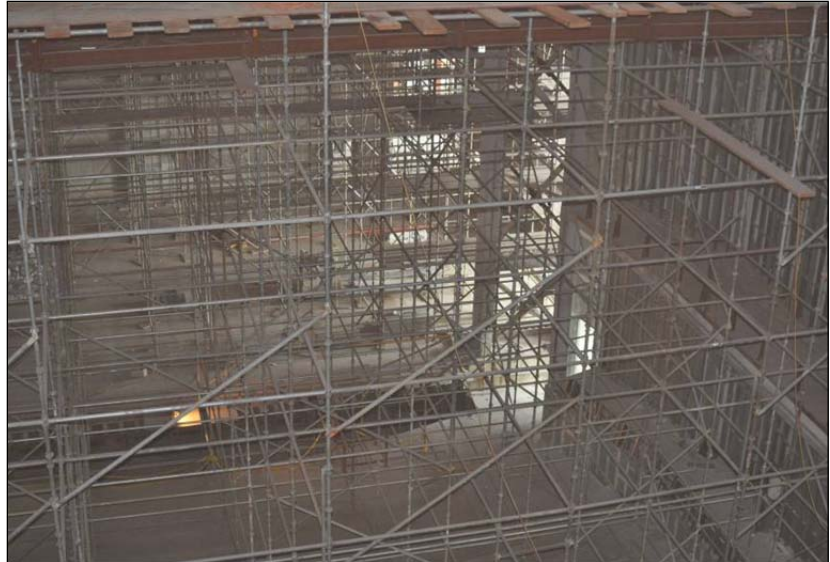
*Picture 8 - Scaffolding in the theater area of the Center, taken February 23, 2011.
