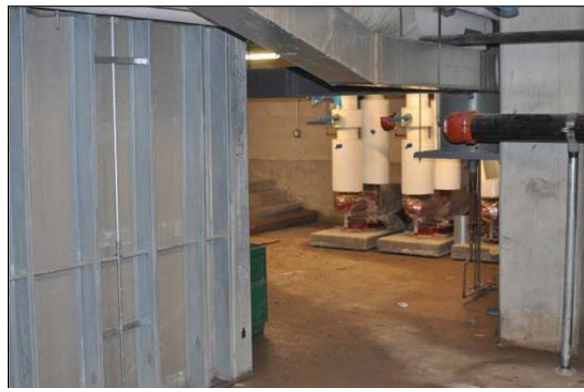
*Picture 4 - Basement area of the Center, taken February 23, 2011.
