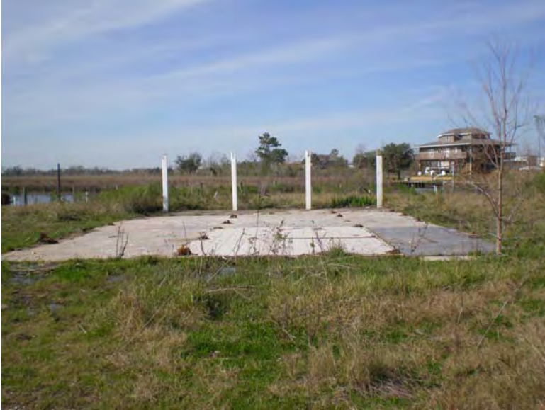
Photo 1: Looking NW towards rear of building footprint
