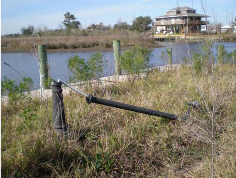
Photo 5: Snapped lightpole
