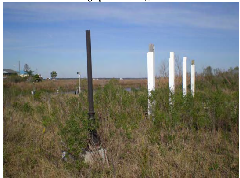
Photo 8: Surviving lightpole and four timber piles
