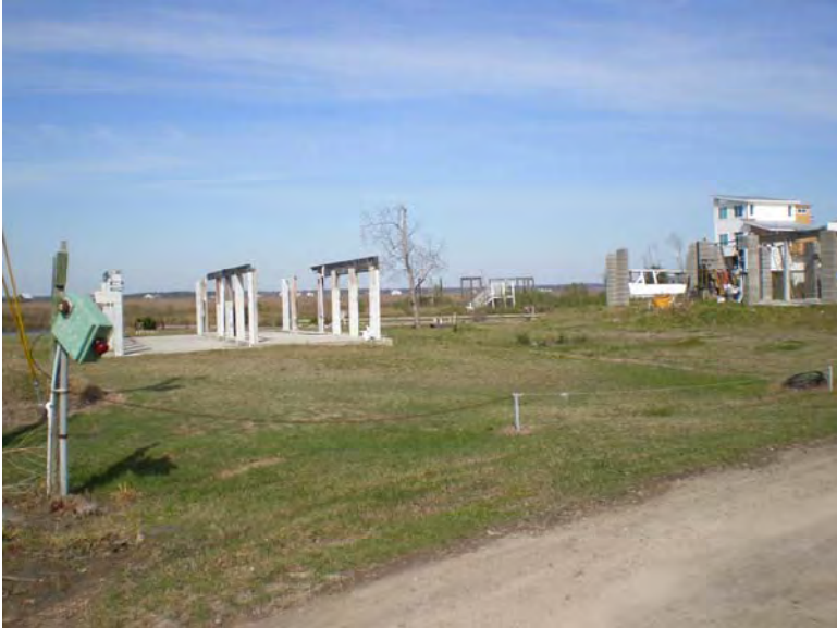
Photo 10: Remaining slabs NE of Anthony residence
