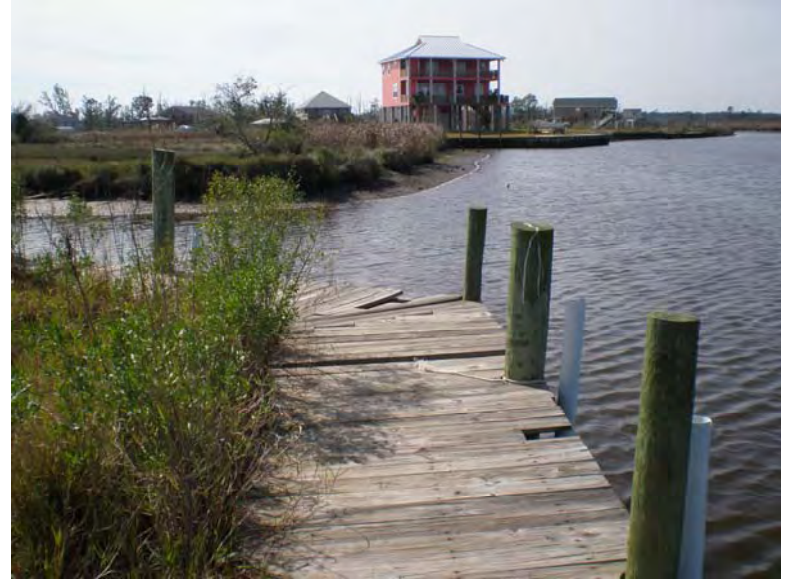
Photo 7: Looking upstream (SW); boat canal at left
