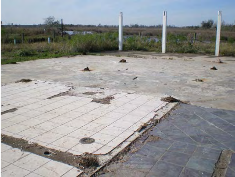
Photo 9: Looking towards rear of building footprint
