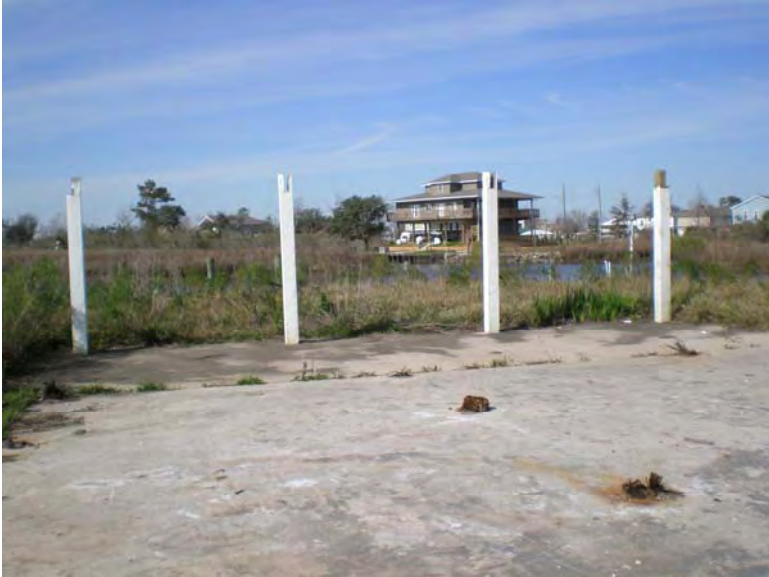
Photo 2: Looking NW towards rear of building footprint
