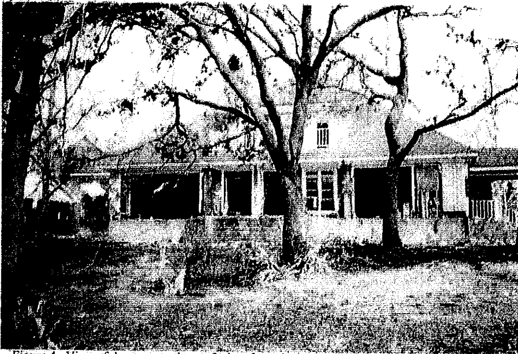
Figure 4. View of damages to the roof taken from the back elevation of the McIntosh Residence
