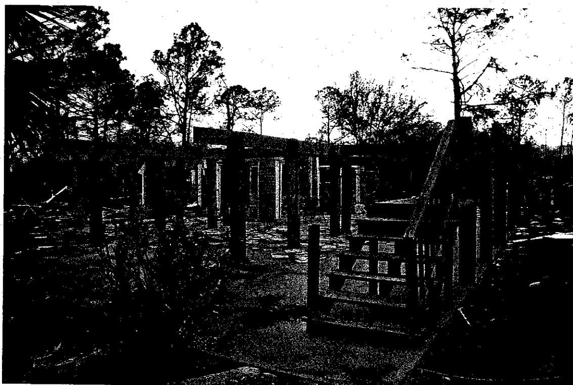
2. Rear elevation view of house.
