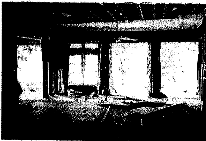
Figure 9. Damage to the interior false ceiling from rain water due to roof failure caused by wind.
