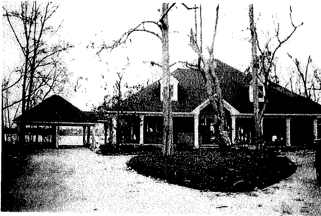
Figure 3. View of the damages to the roof taken from the front elevation of the McIntosh Residence
