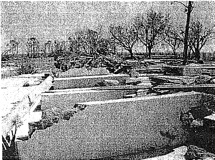
Slab and debris
