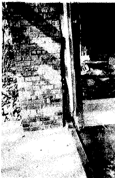
Figure 14. Horizontal shear cracking of column encasement and separation from the house envelope.
