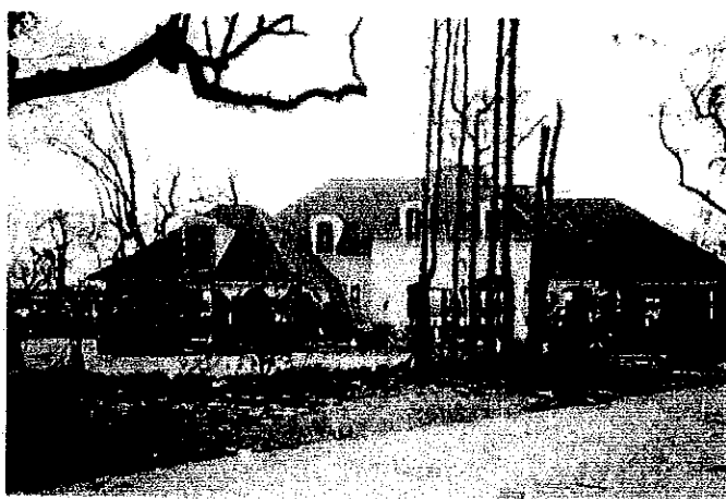
Figure 11. Trees in the yard stripped and broken due to high wind velocity.
