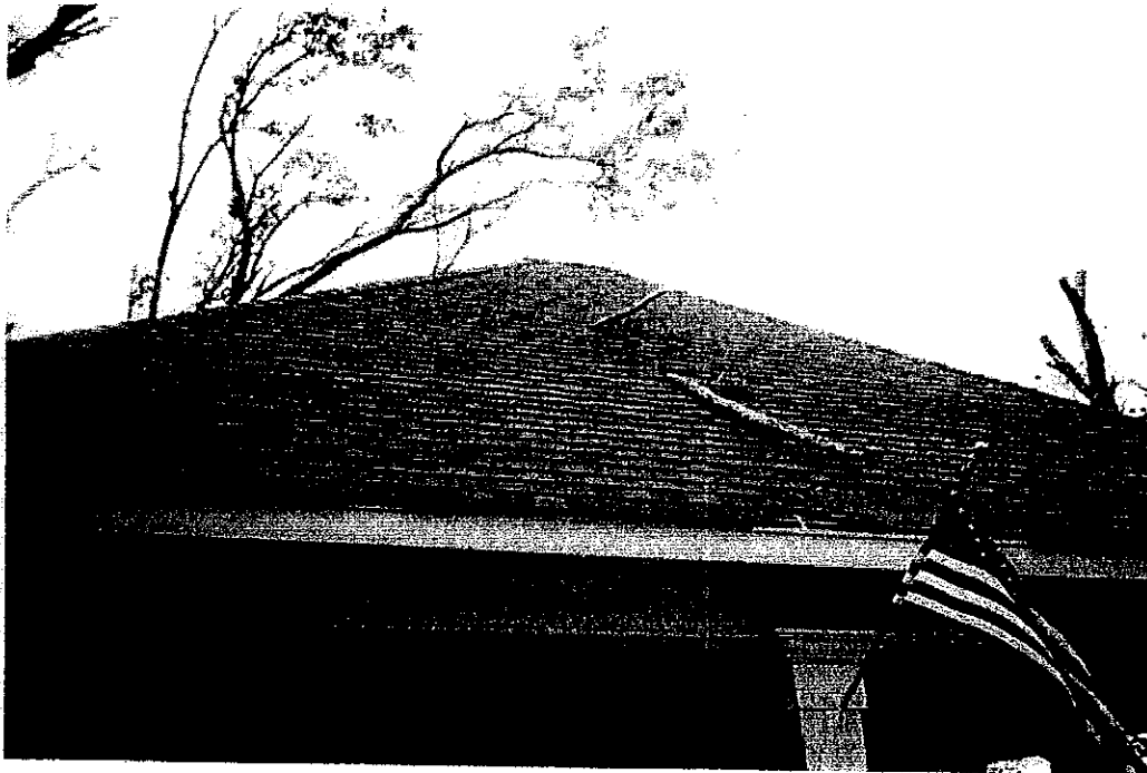
Figure 5. View of uplift damages and penetration of debris to the McIntosh roof
